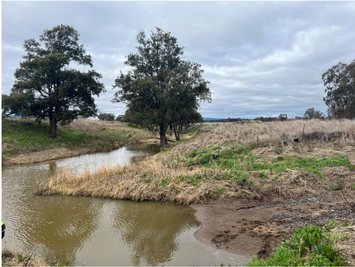
Photo 3 – Oakey Creek Causeway, Neible Siding Road, Coolah – 25 August 2022 – Looking upstream
