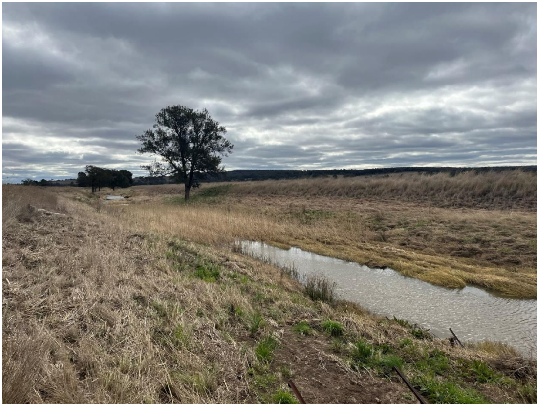
Photo 2 – Oakey Creek Causeway, Neible Siding Road, Coolah – 25 August 2022 – Looking downstream
